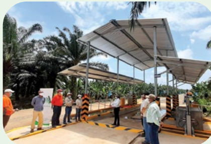
Foot bath and tire bath for Fusarium TR4 prevention through the disinfection of vehicles and hygiene at the entrance of people
